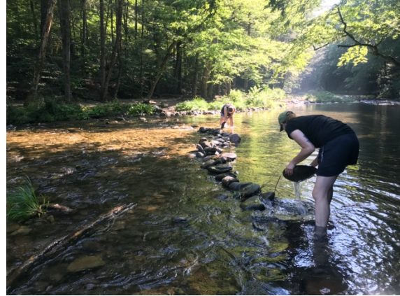
Figure 7: Anna and Jenny dismantle a visitor built rock dam in the Rondout Creek
