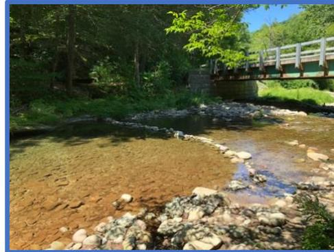
*Figure 14: One of the largest rock dams found, this dam raised the upstream level by 3.5"*
