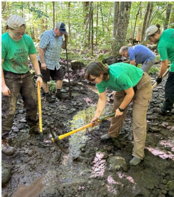
Stewards digging drainage in Sundown Wild Forest
