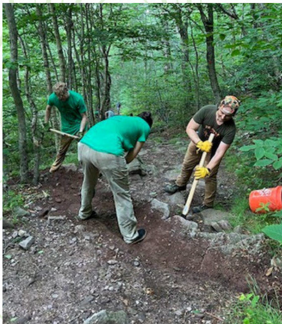
One of the water bars being cleared on Slide Mtn
