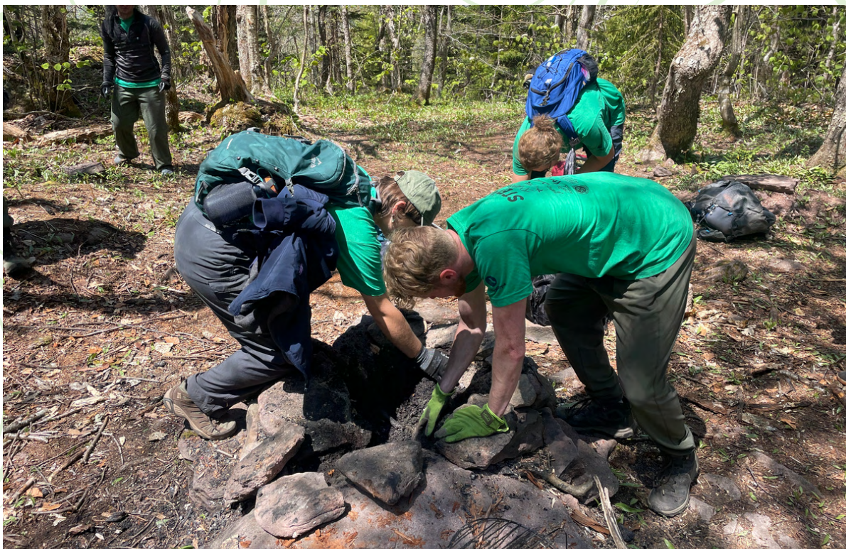
The stewards cleaning up and rebuilding a designated fire ring at one of the Giant Ledge campsites
